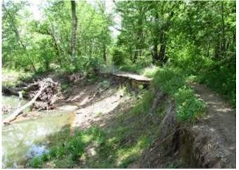
Failed Trail Due to Stream Bank Erosion
